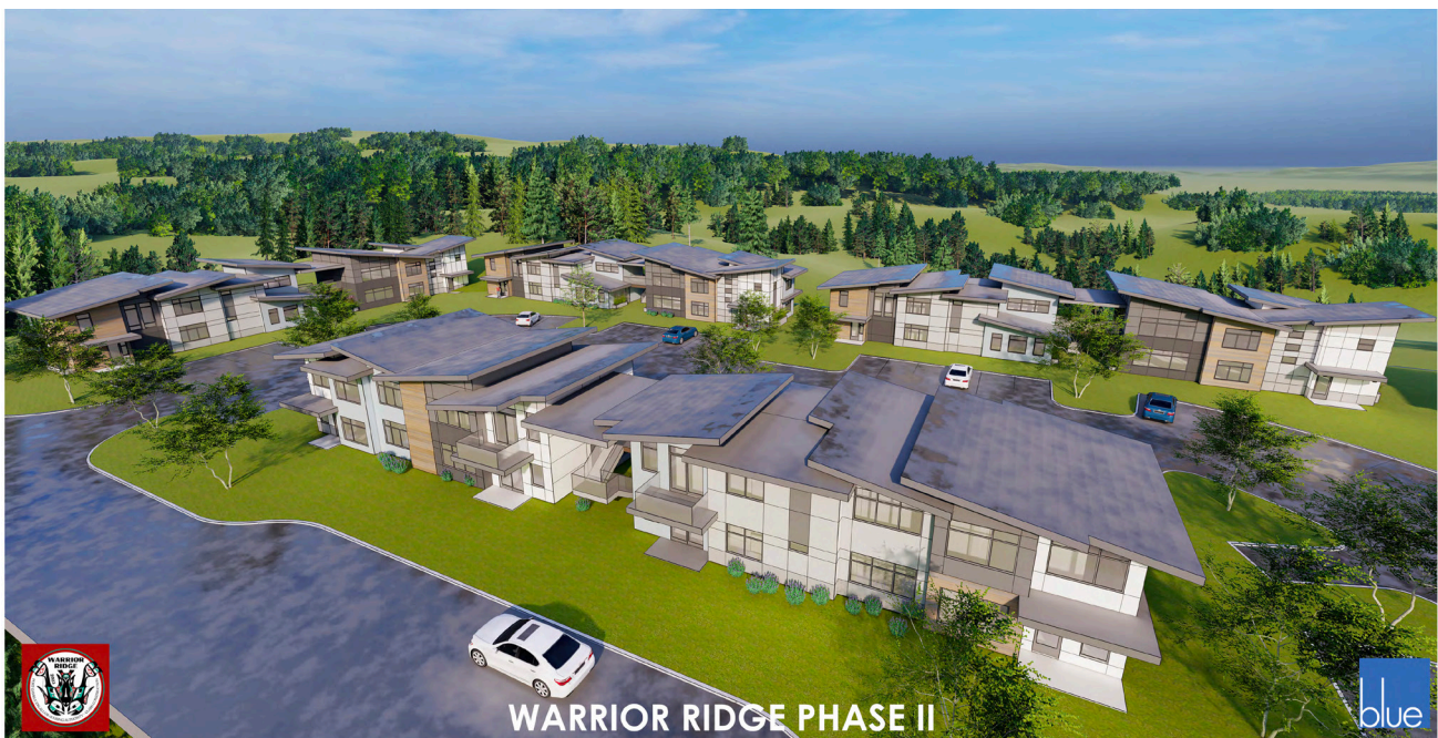
Below: A rendering of Phase II of Warrior Ridge, which is currently under construction
